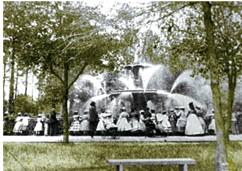
Fig. 40 | Water fountain at Forsyth Place (Park), circa. 1868 (Unknown, n.d., edited by author)
