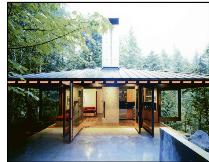
▲ Figure 21 (Olson Kundig Architects, n.d.) overlay by author The strong roof line acts as a datum gathering spaces below.
