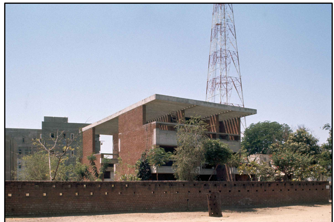
▲ Figure 10 (Serenyi, 1975) overlay by author Overhead pergola and recessed terraces proved shade for exterior and interior spaces. landscaping further protects against solar gain. The building's materials of brick and concrete can both be locally sourced and erected.
