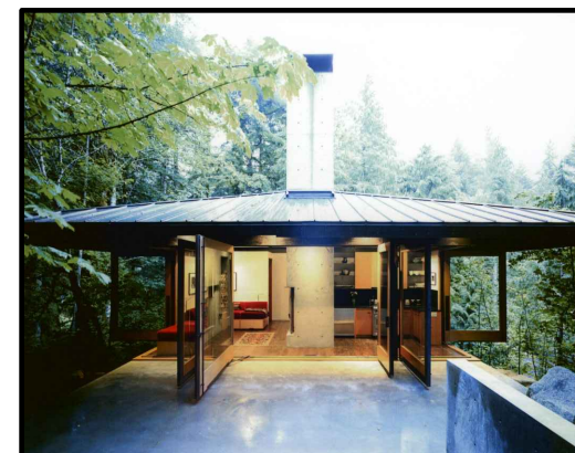
▲ Figure 33 (Olson Kundig Architects, n.d.) Large overhangs provide shade to the interior of Tye River Cabin while the surrounding trees help diffuse the low direct sun from east and west.
