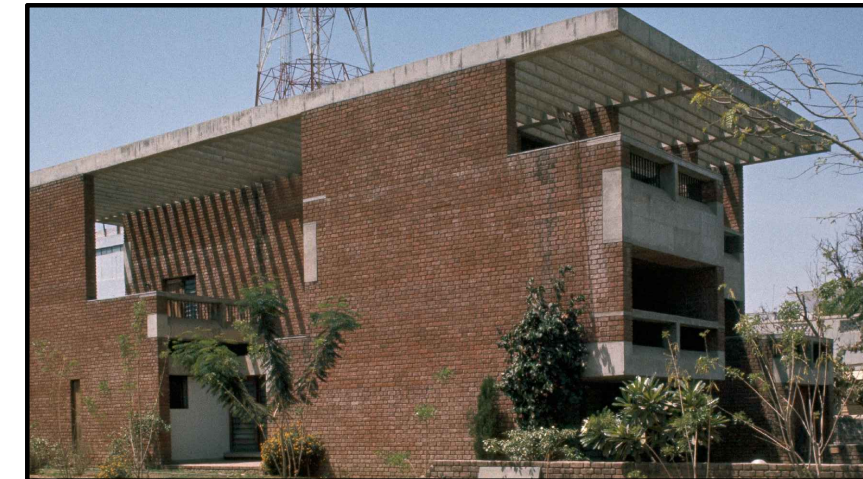
▲ Figure 34 (Serenyi, 1975) Concrete and brick provide thermal mass at Parekh House, dampening the transfer of heat to the buildings interior.
