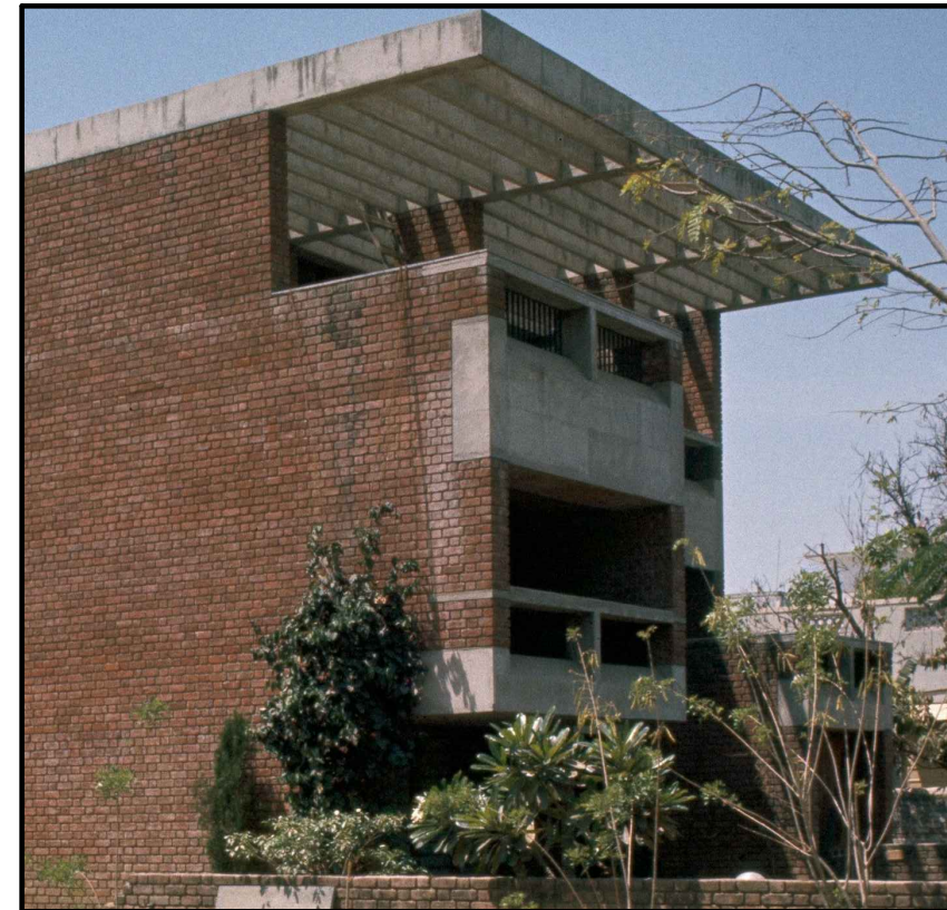
▲ Figure 44 (Serenyi, 1975) Brick and concrete can be locally sourced and installed at Parekh House and provide a durable, low maintenance finish.
