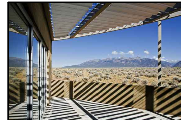
▲ Figure 31 (Serenyi, 1975) An overhead pergola helps to shade Parekh House from the high sun.
