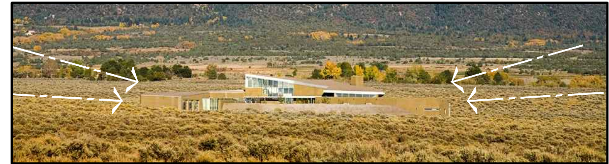
▲ Figure 41 (Antoine Predock Architect, n.d.) Limited openings are located on the east and west elevations of Sage House due to low sun angles from these directions.
