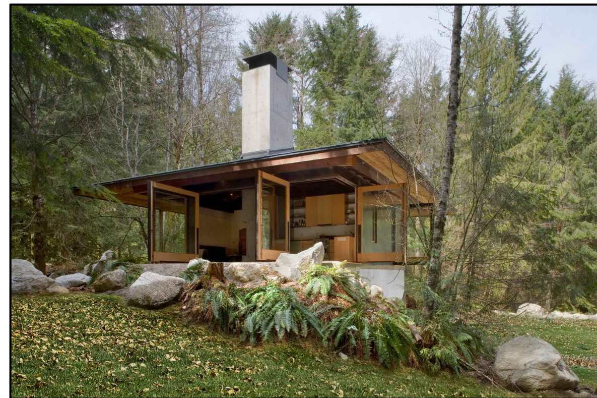
▲ Figure 17 (Olson Kundig Architects, n.d.) Tye River Cabin.
